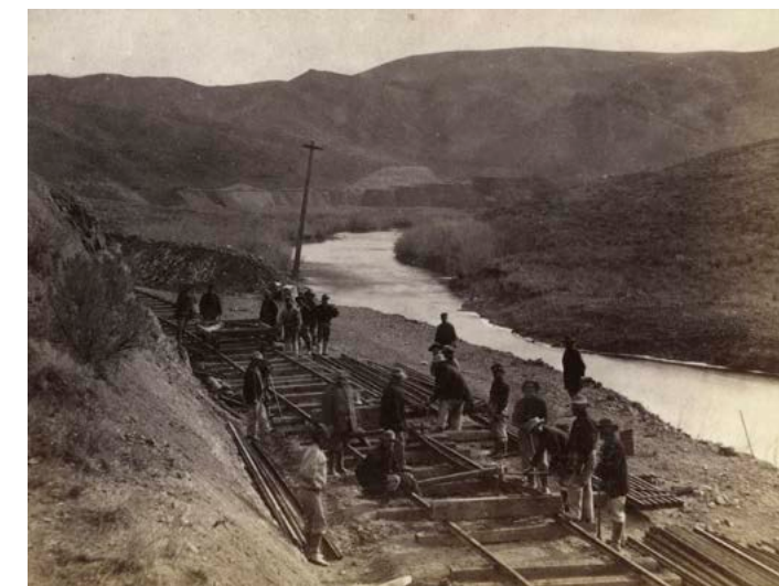
Workers lay track along the Ten Mile Canyon (Image Credit: Alfred A. Hart Photographs, 1862-1869, Department of Special Collections, Stanford University Libraries).
